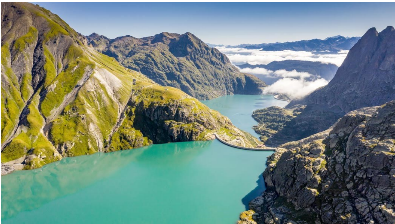
Nant de Drance pumped storage power station in the Valais Alps. View on the Vieux Emosson reservoir, 295 meters below is the Lac d'Emosson. Photo: Sébastien Moret
