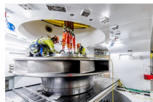
Assembling a pump turbine.
