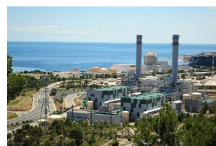
Plana del Vent gas-fired combined cycle power plant in Spain.
