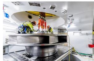
Assembling a pump turbine.
