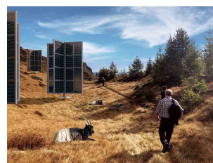
Solar trees from the Gondosolar PV project in Valais.
