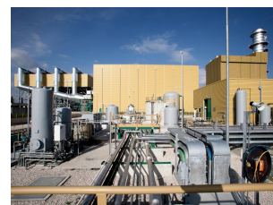
The San Severo gas-fired combined-cycle power plant is comprehensively modernised.
