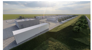
Alpiq is investing in new battery projects in Finland and France.
